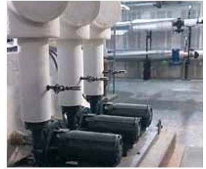
Pictured at top: High Rise Building, Mexico City, MX. Pictured in the middle and at bottom: Texas Children's Hospital, Houston, TX.
